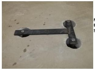
Note: Anchor must be Electrically bonded. Please See the NEC requirements.
