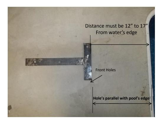
**STEP 1**: Locate the retro-fit anchoring system template (included and shown above)
