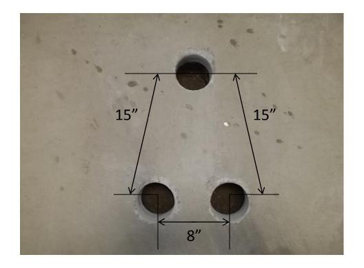
**Step 2**: You will need a 4" diameter core drilling bit.
